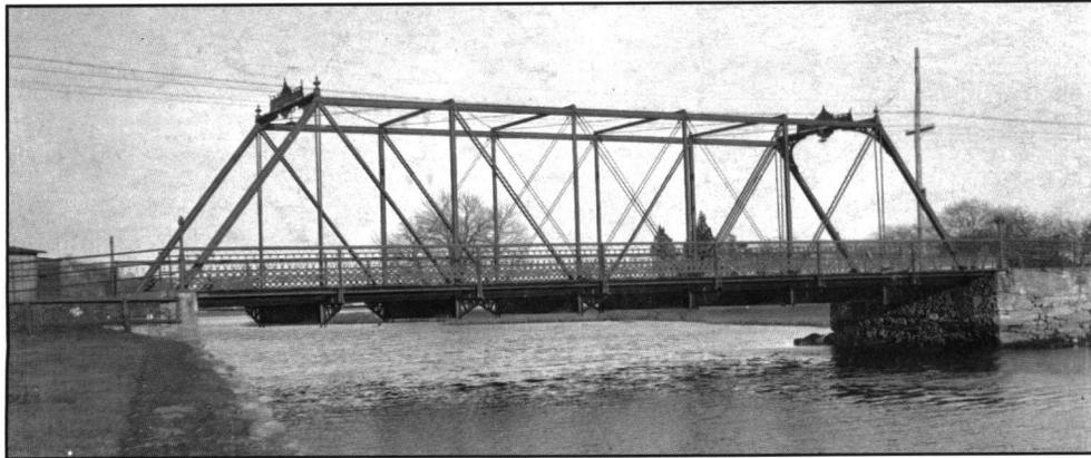
*Starting in 1913, the State began replacing the iron trusses of the 1880s with concrete bridges. This truss in Wickford was replaced with a concrete arch in 1925.*
